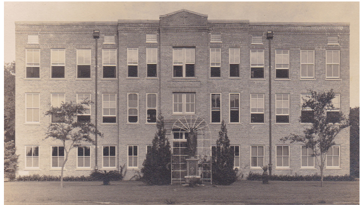
Minor Seminary Building Dedicated September 16, 2023
